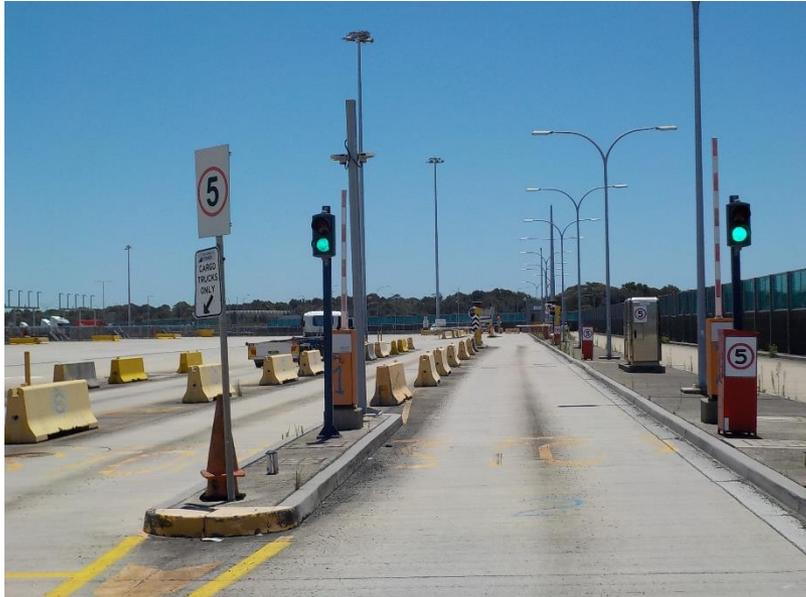
All trucks exiting the Terminal is subject to Weigh in Motion (W.I.M). This will provide a weight of the vehicle as well as a height reading to comply with the appropriate regulations.
